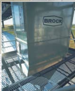
Optional enclosed gravity belt take-up
