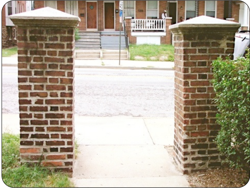
Repaired Columns in York Court 2
