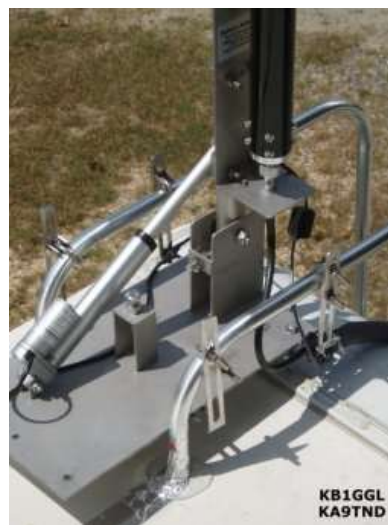
Picture 4 – MT-1 & Automatic Lift & Lay
