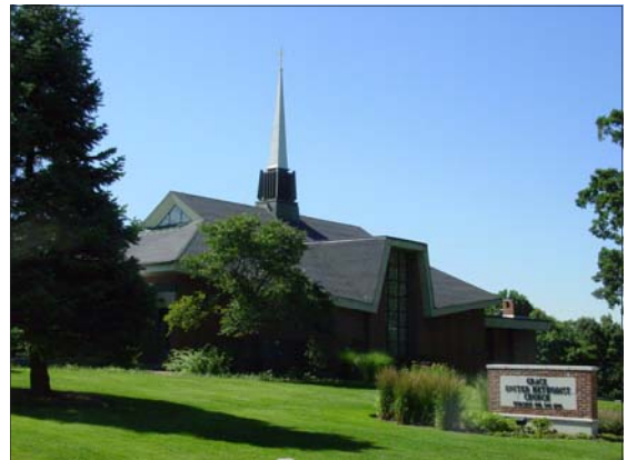
Among other responsibilities, the Grace Board of Trustees makes sure our building is at its best.
