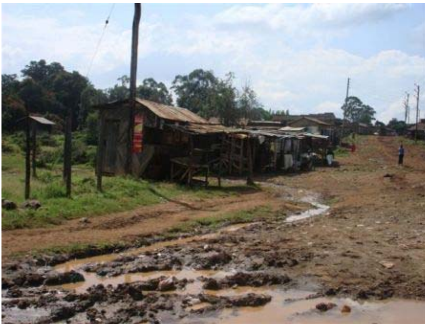
Yes, this is the town of Kabimoi where The Harvest Church is located. The town is very small and very poor. However, the church family is so excited about their new church - and the new bathroom facilities next to it! God is good and at work in this place!
