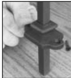
The C-2910 Flared Collar with Screws is an installation system where the drilling of treads is not required. Trim the baluster flush to the top of the tread....
