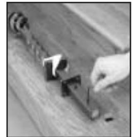
1. Begin installation by drilling or cutting a hole in the proper location. With the base collar placed on the newel, attach the shaft to the pre-cut newel with the provided allen wrench and screws.
