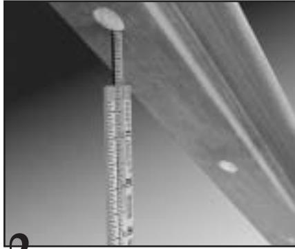
**2.** With all baluster holes drilled and the rail temporarily set back in place, use a carpenter's rule to measure the exact distance from the tread to the lower side of the drilled  $1/2''$  diameter hole in the rail.
