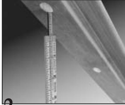
**2.** With all baluster holes drilled and the rail permanently installed, use a carpenter's rule to measure the exact distance from the tread to the lower side of the drilled  $1/2''$  diameter hole in the rail.
