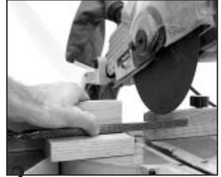
**3.** After adding  $1/2''$  for insertion into the rail and  $3/8''$  for insertion into the tread (a total of  $7/8''$ ), use a chop saw equipped with a standard  $1/8''$  flexible cut-off blade to trim the baluster to the exact length.
