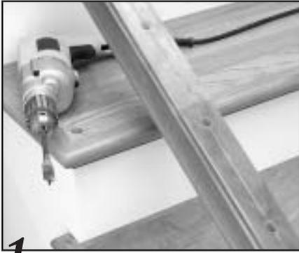
**1.** Begin the installation by **TEMPORARILY** attaching the handrail throughout the stair and marking the treads and underside of the rail for baluster placement. At each baluster location drill the appropriate diameter hole  $3/4''$  deep into the treads and a  $1/2''$  diameter hole approximately  $1''$  deep in the underside of the rail.
