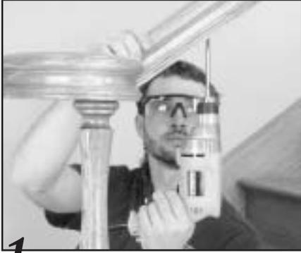
**1.** Begin the installation by **PERMANENTLY** attaching the handrail throughout the stair and marking the treads and the underside of the rail for baluster placement. At each baluster location drill the appropriate diameter hole  $3/8''$  deep into the treads and a  $1/2''$  diameter hole approximately  $1''$  deep in the underside of the rail.
