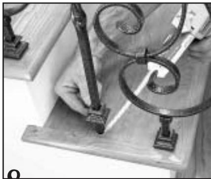
**8.** Finish the installation by using epoxy to fill any void around the base of the baluster and to secure the Base Collar.
