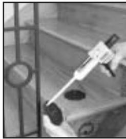
Medallions consist of two halves that screw together. Apply epoxy adhesive on the screw and contact points....
