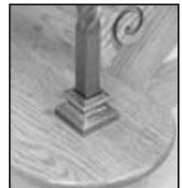
3. Finish the installation by using epoxy to secure the base collar.
