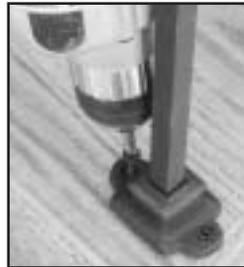
...and secure the base collar by predrilling and screwing into place.
