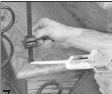
**7.** Finish installation by using epoxy to fill any void around the base of the baluster and to secure the base collar.
