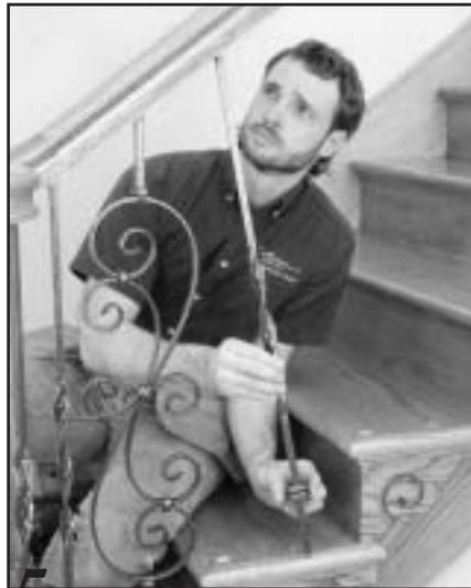
**5.** With the base collar placed on the bottom of the baluster, work the baluster into place by inserting the top of the baluster into the rail hole and sliding the bottom of the baluster over and down into the tread hole.
