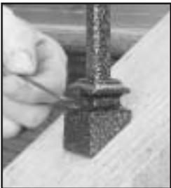
Rake Collars (*angled collars*) replace the base collar on knee wall stairs. Place a collar onto the bottom of all balusters before installing. With the collar resting firmly on the knee wall, permanently attach the rake collars by tightening the provided set screw.
