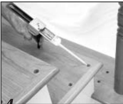
**4.** When all balusters are trimmed, remove the rail from the newels and deposit epoxy adhesive into each baluster hole in both the treads and the rail.
