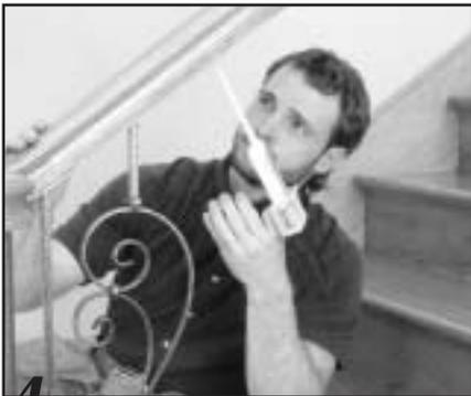
**4.** Working one baluster at a time, deposit epoxy adhesive for a single baluster into both the tread and baluster hole.
