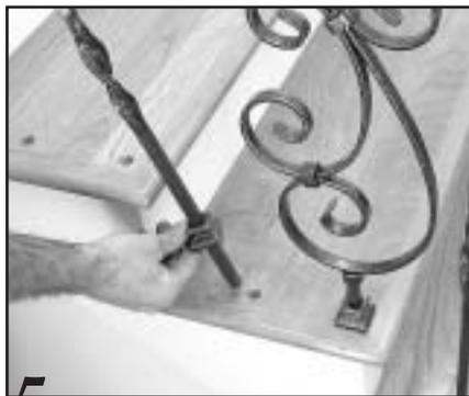
**5.** With the base collar in place on the bottom of the baluster, set each baluster into the tread hole.
