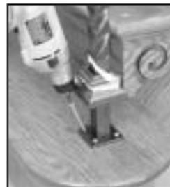
2. Place the shaft into the hole and permanently attach with provided 3" anchoring screws.
