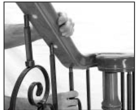
**6.** Working one baluster in at a time, replace the rail system on top of the balusters and install the rail permanently to the newels.
